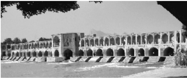
The Khajou Bridge during daylight.
